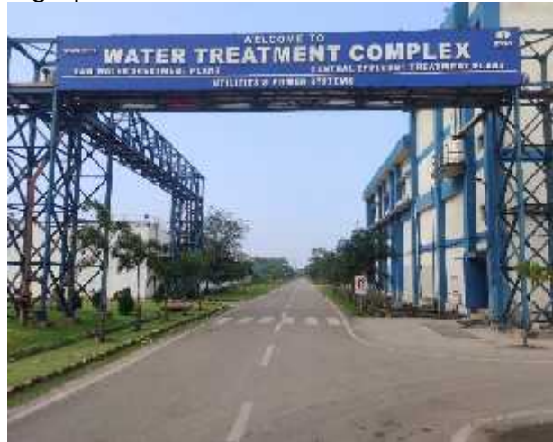
Water Treatment Complex (RWTP and CETP)
