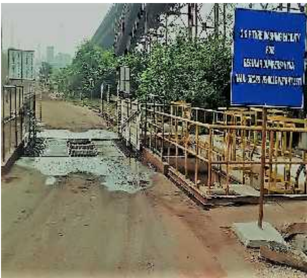
Wheel Washing facility at Ore & Flux Yard
