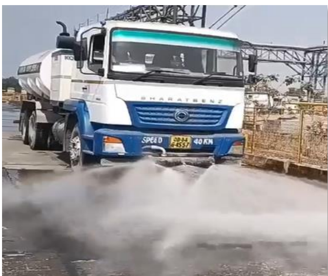
Mist type water sprinkler
