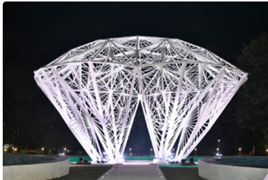
Jamshedpur's Jubilee Diamond at Dorabji Tata Park in Jamshedpur, built using Tata Structura Steel Hollow Sections
