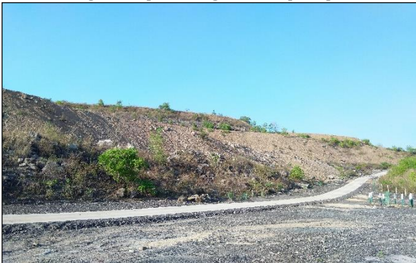
Soil & grass Spreading on dump slope
