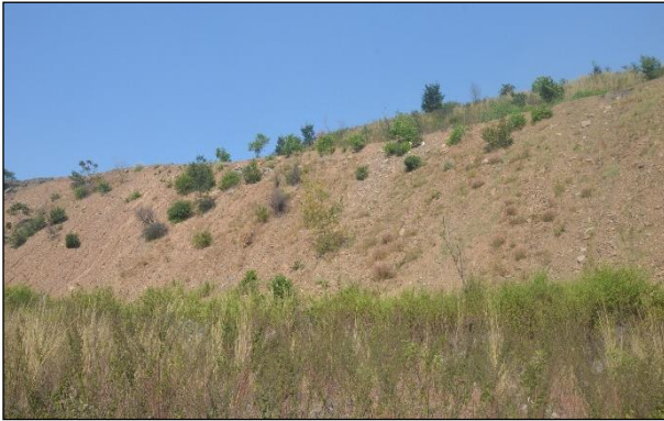
Soil & grass seed Spreading on dump slope
