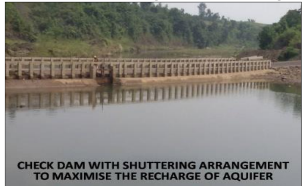
Check Dam to increase ground water recharge
