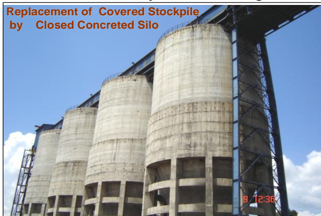
Concrete silos for material storage
