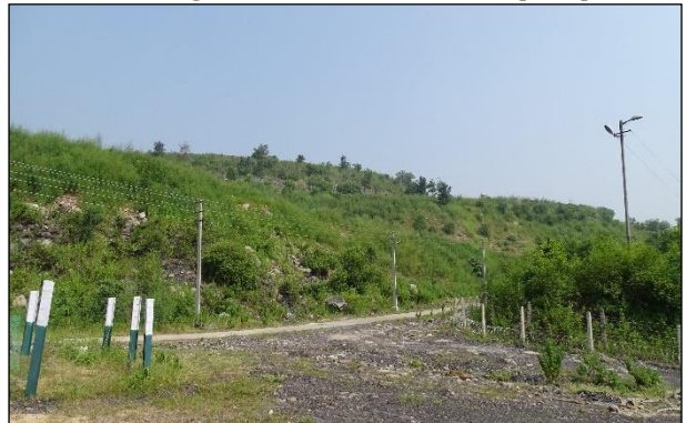
Grassing and Plantation on dump slope
