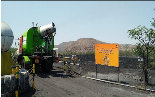
Water Mist Canon in coal stacking area
