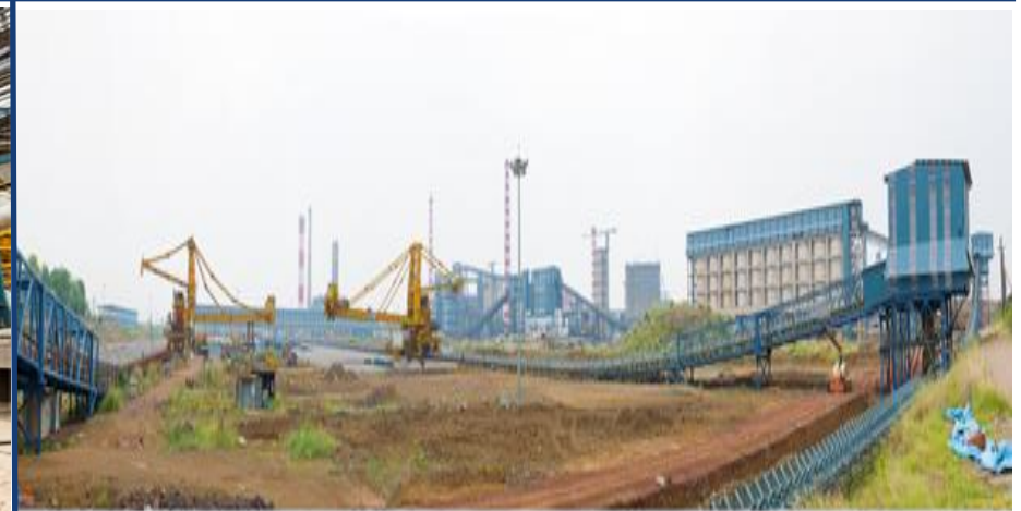
Raw Material Handling System Conveyor Belt
