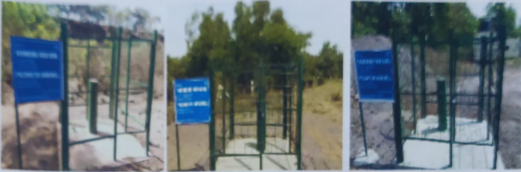
Piezometer (PB gate, Garden area, N orebody area)
