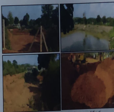
Four number of ponds being modified
