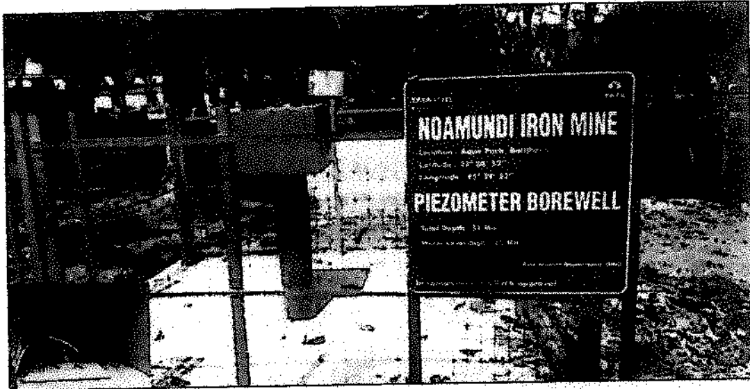
Piezometric borewell installed at Aqua Park, Noamundi Mine
